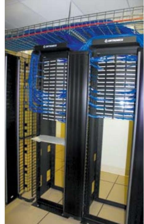
**Berk-Tek’s Augmented Category 6 cable runs neatly overhead in the Cablofil wire mesh tray and is neatly terminated into the switch patching fields in the Ortronics’ Mighty Mo racks.**
