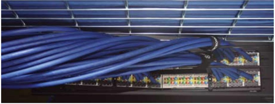
**Pictured are two Ortronics' stacked overhead patch panels, offering a flexible solution and reducing valuable space within the racks and cabinets.**
