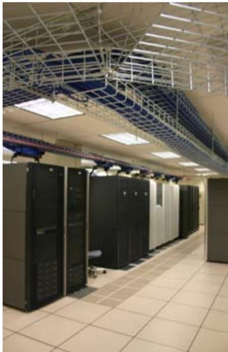
**The rows of cabinets and racks are aligned in a hot/aisle cold/aisle scenario, connected with overhead Augmented Category 6 cable in the wire mesh basket. This layout is considered as one of the best practices in the TIA-942 data center standard.**
