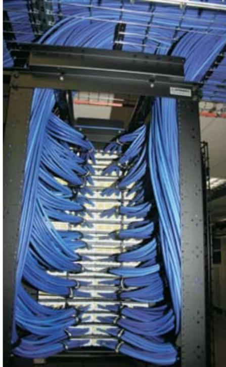
**Berk-Tek’s LANmark-10G Augmented Category 6 cable is neatly managed, dressed and terminated in the Ortronics’ patch panels in the rack.**
