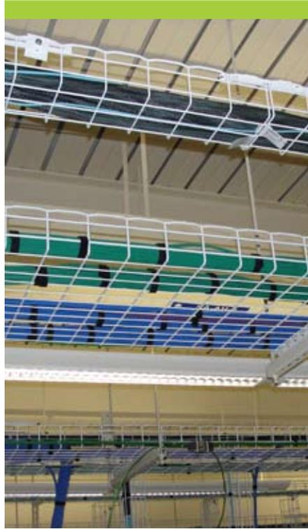
The TIA-1179 standard brings attention to separating cables by application, as shown here in the new Tifton Medical Center.
