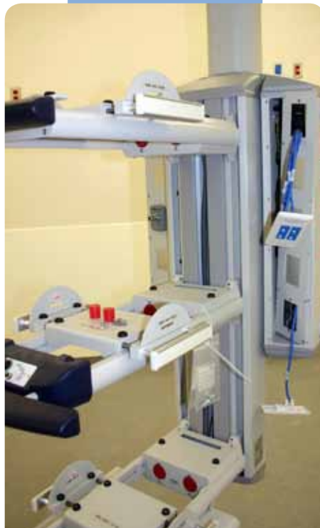
The right cable should be matched to the environment. For example, the operating room booms require a flexible network cable.
