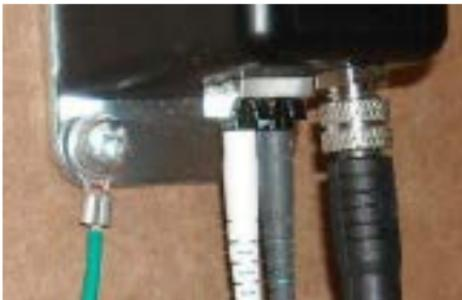
The installer must mount the OneReach units such that the base plates are connected to local ground. This is done by using grounding screws (not supplied) to secure the metal base of the PI source or remote to a mounting plate connected to an approved ground.
